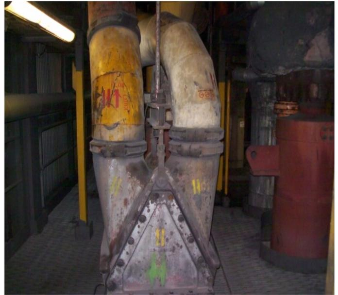
Figure 5. A riffle box divides a fuel pipe into 2 burner pipes.
