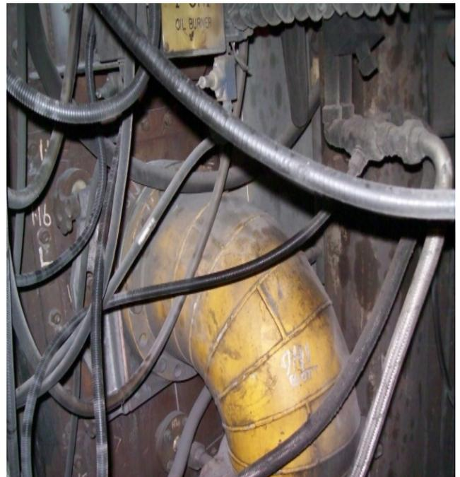
Figure 6. A 12" (305mm) burner pipe delivers pulverised coal to a boiler's furnace.
