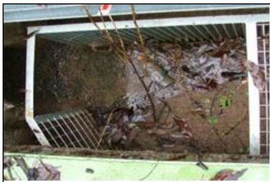
Figure 8. A snapshot of a field investigated GPT showing deposits of sediments which are similar to the pattern from the gross pollutant capture/retention experiments with partially buoyant spheres (See figure 7). Note the blocked inlets in both cases.
