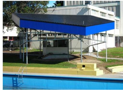
Figure 5: Building integrated solar collector for heating diving pool
