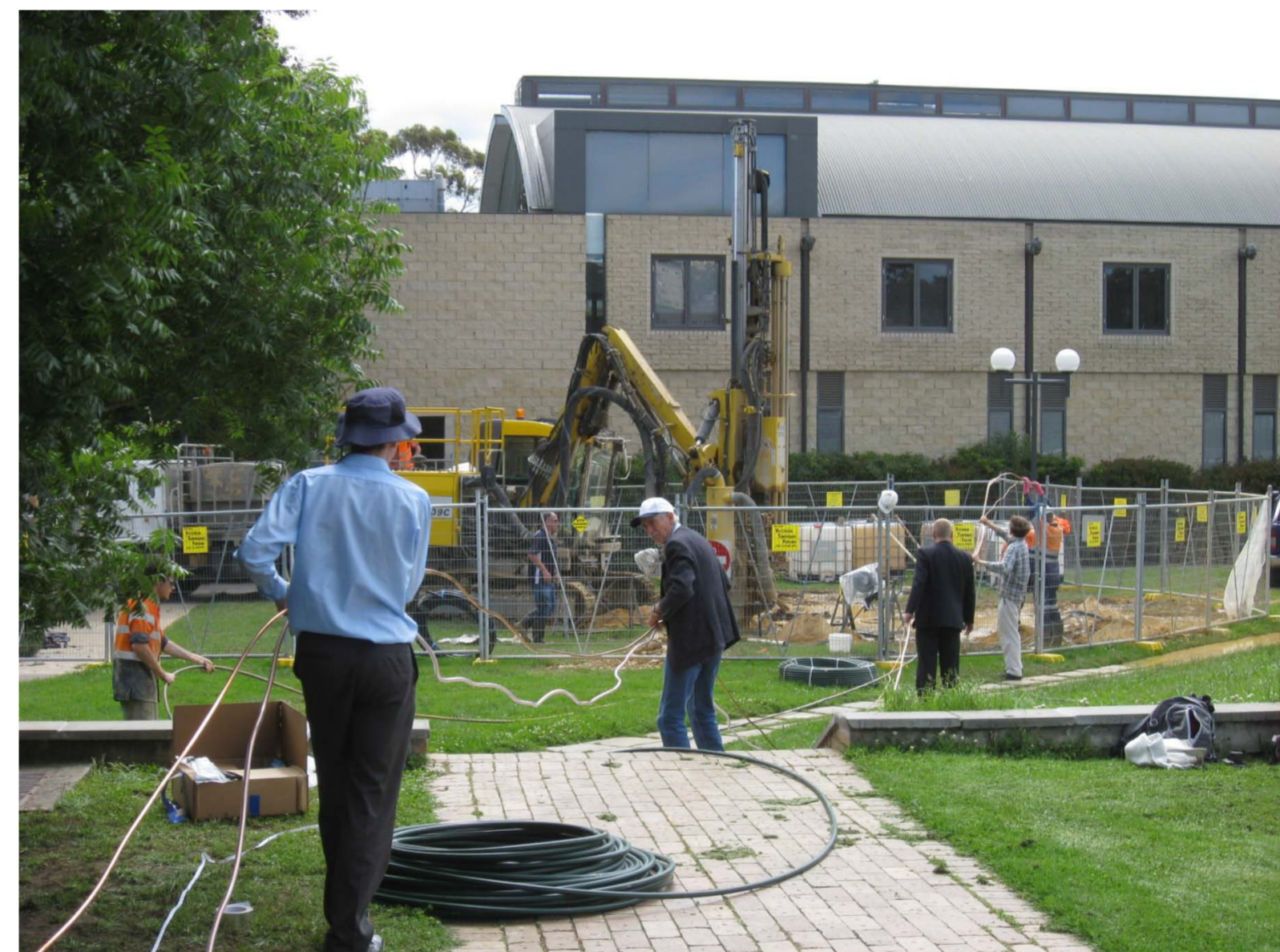
Left: Copper loops, through which refrigerant will circulate as part of a direct exchange system, are lowered into a 30m deep borehole
