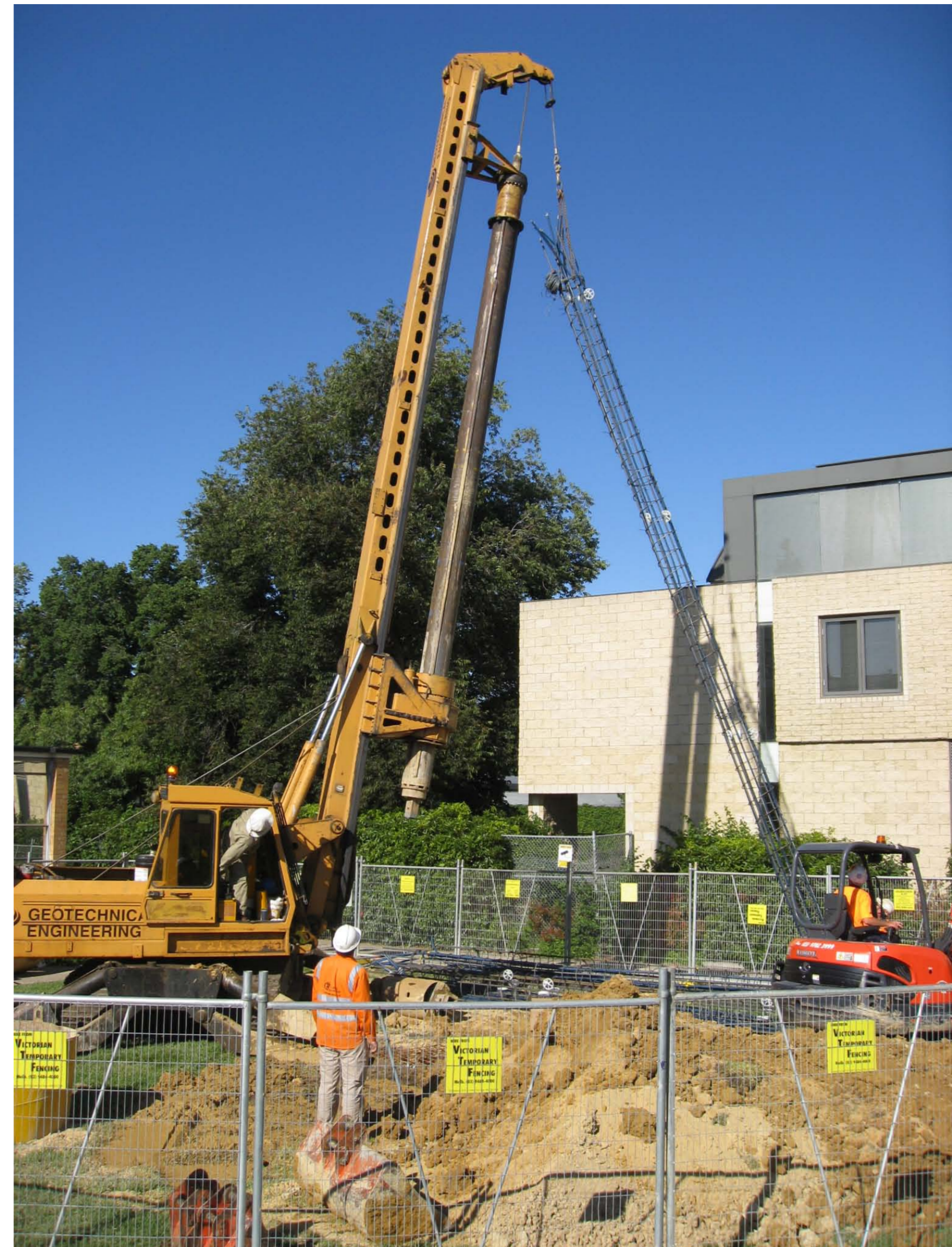
Left: A section of reinforcement cage (with piping attached) is lifted before being lowered into a 30m deep energy pile
