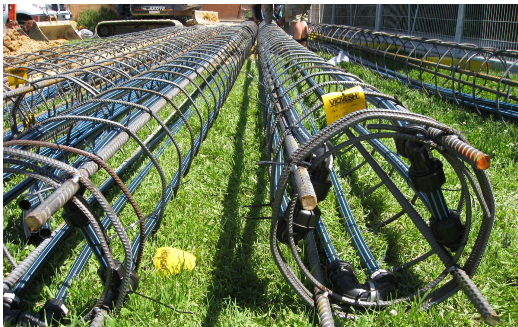
Left: The primary circuit of an energy pile comprises HDPE pipes attached to a steel reinforcement cage. Water will circulate through the pipes
