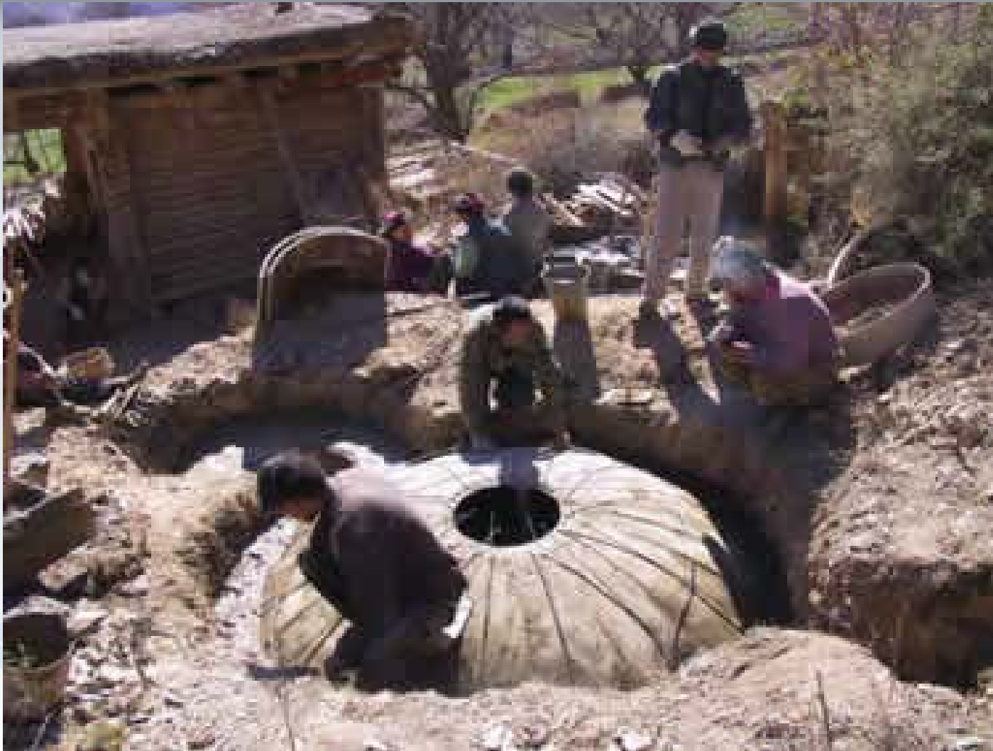
A rural biogas plant under construction (Usher & Wang 2002)
