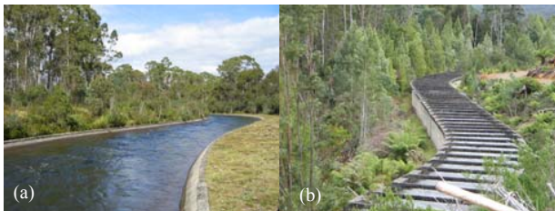
Figure 1. Tarraleah No.1 Canal (a) Trapezoidal in-ground canal section. (b) Rectangular above-ground flume section.
